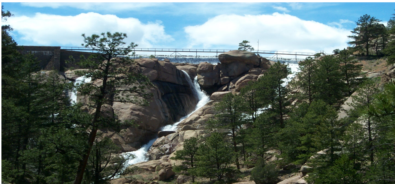
A 21st Century picture of Cheesman Dam spilling to the South Platte, taken in 2005 showing some recovery from the Hayman Fire.
